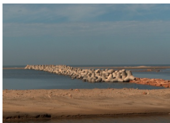
Figure 2: Sea revetment structure where offshore mariculture system will be deigned to protect from erosion
